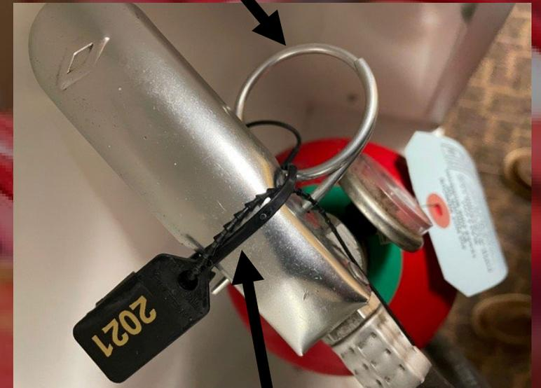
**SEAL** - KEEPS THE PIN IN PLACE
